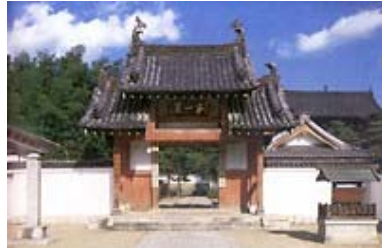
Main Entrance Gate
